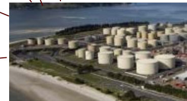
Distribution terminal facilities
