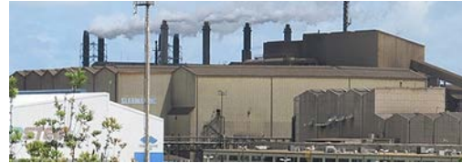
Glenbrook steel mill co-gen
